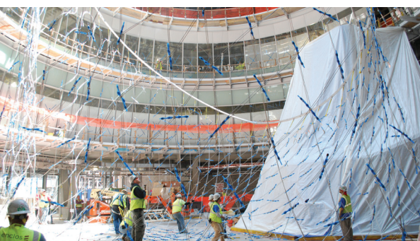
^ SEQUENCE 2 The installation sequence of the double-curved cable structure with universal paddle-connectors pre-located within the tight, enclosed confines of the project site. The sequence includes the arrival of the net as a single piece, which was then attached to the ring beam and hoisted with a high precision lift to avoid damaging already installed structures. The entire installation of the net from the truck to a hanging position was done in one day, using one lift.
