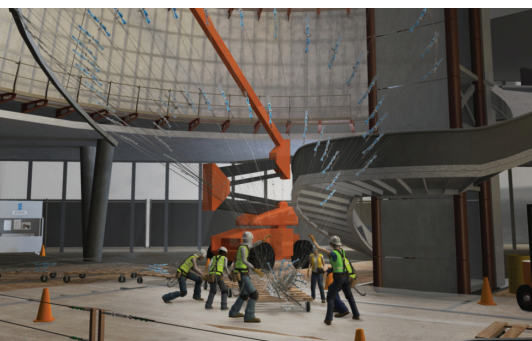
^ SEQUENCE 1 Animated installation sequence used to educate field crews on installation and safety tactics. Additionally, lifts of large objects through small spaces were studied to ensure proper clearance in the field.
