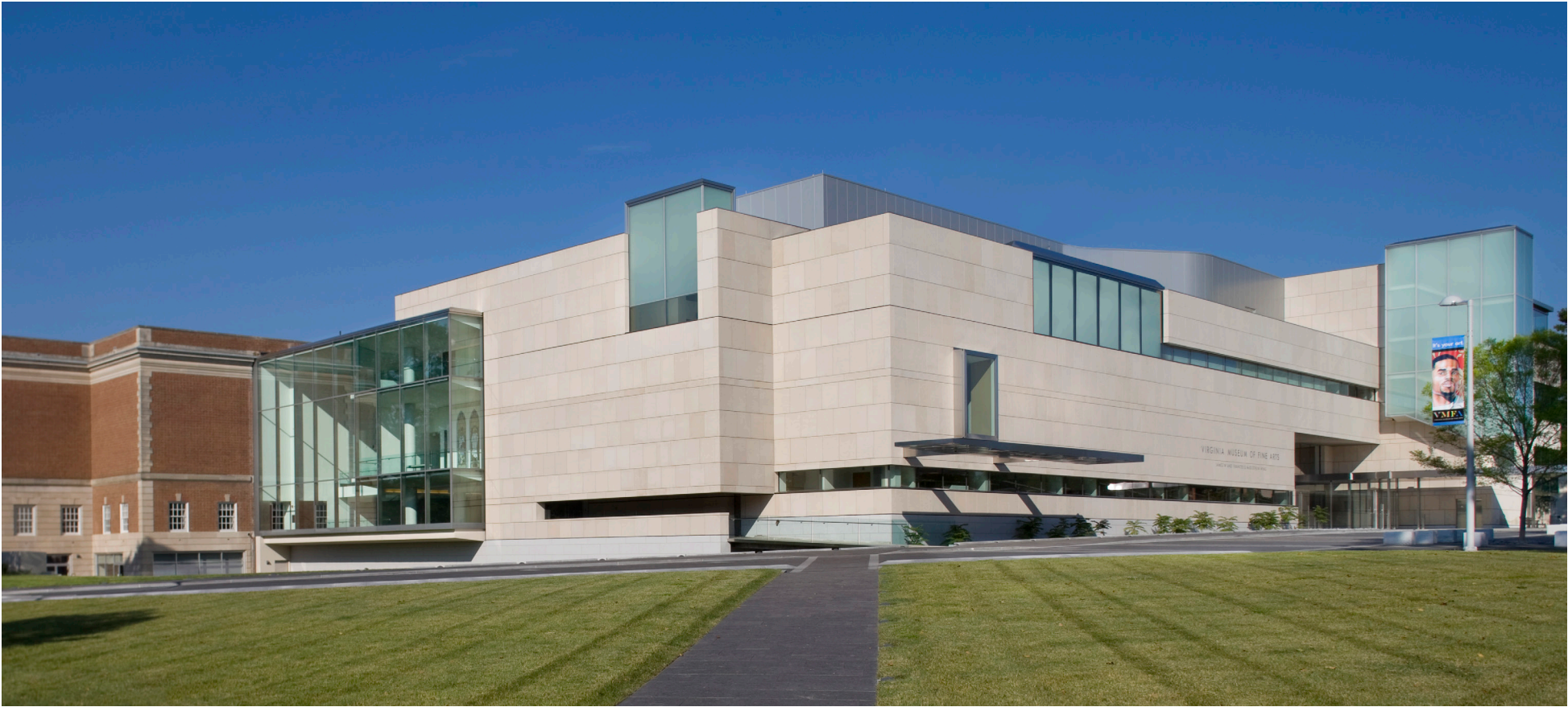
Figure 1: The McGlothlin wing uses Indiana limestone to blend the new building structure with the existing 1936 structure. Image by Bilyana Dimitrova, courtesy of Virginia Museum of Fine Arts.
