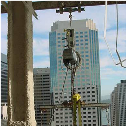
Monorail Installation Method
