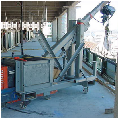
Floor Crane Installation Method
