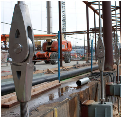
Figure 8. Construction photos; soffit (left) and bottom cable connection (right).
