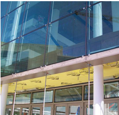
Figure 8. Construction photos; soffit (left) and bottom cable connection (right).
