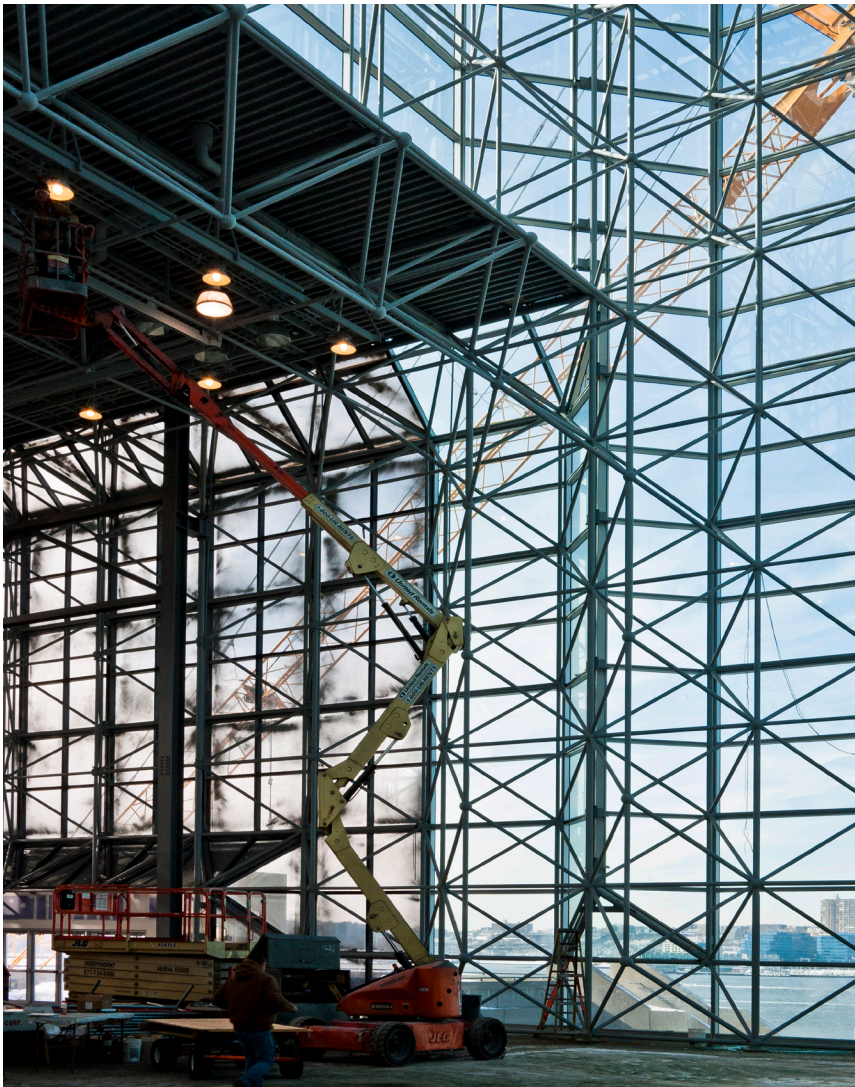
Figure 8: The Javits Convention Center in New York City is currently undergoing a facade retrofit involving the removal and replacement of the entire facade system.
