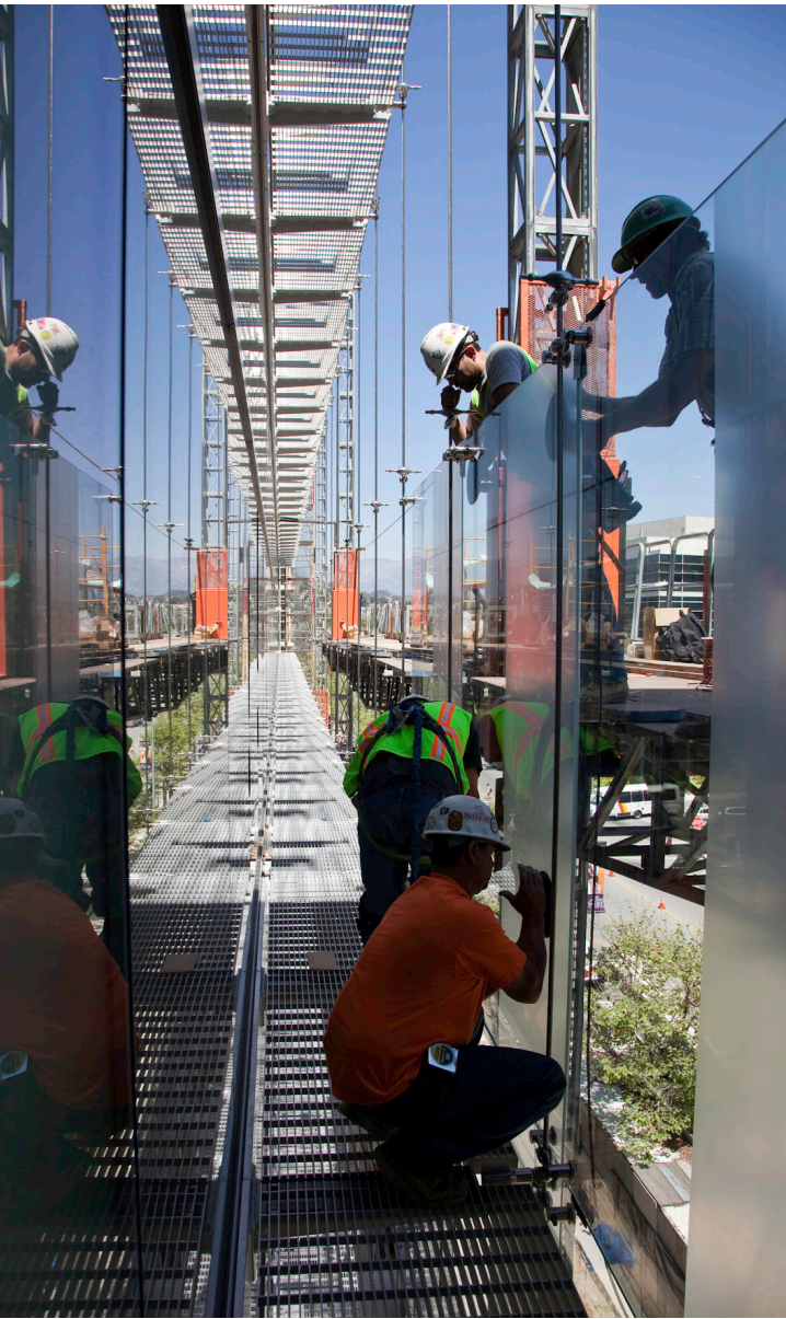
Figure 5 (above): Working within the deep cavity of a multi-story double skin system, workers install the outboard skin. A grating system divides the cavity at each floor level to provide maintenance access without restricting airflow.
