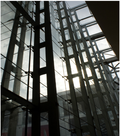
Figure 1. LA Live Podium AESS trusses.
