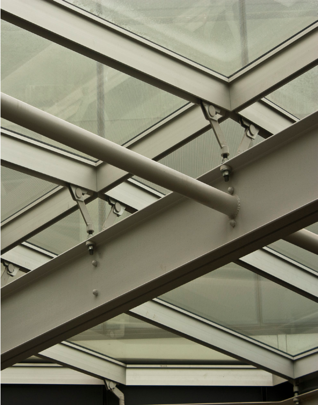
Figure 6: The skylight framing is supported by perimeter building structure and the dramatic yellow “tree” truss which houses central circulation.
