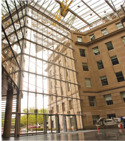
Figure 3: Atrium entrance wall with vertical and horizontal springs.
