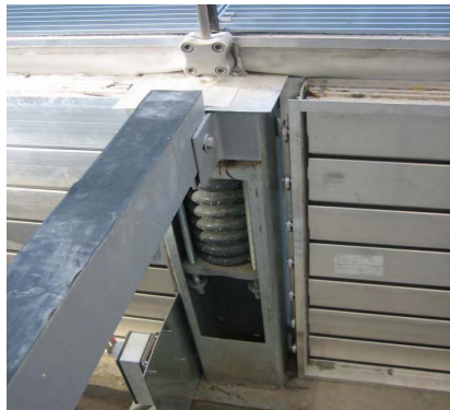
Figure 8: Detail of the vertical cable base spring connection. This keeps the system in tension while allowing for cable deflections under load.
