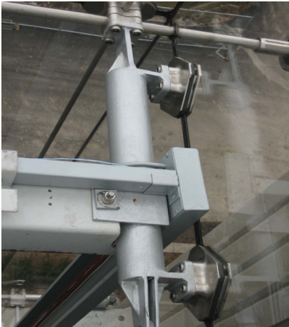
Figure 10: Horizontal cable penetration through the glass. The vertical rail below is part of the motorized blind system.
