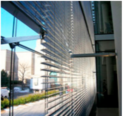
Figure 1 (top left). Mock-up of 5-in deep double-skin box windows placed within a unit assembly.
